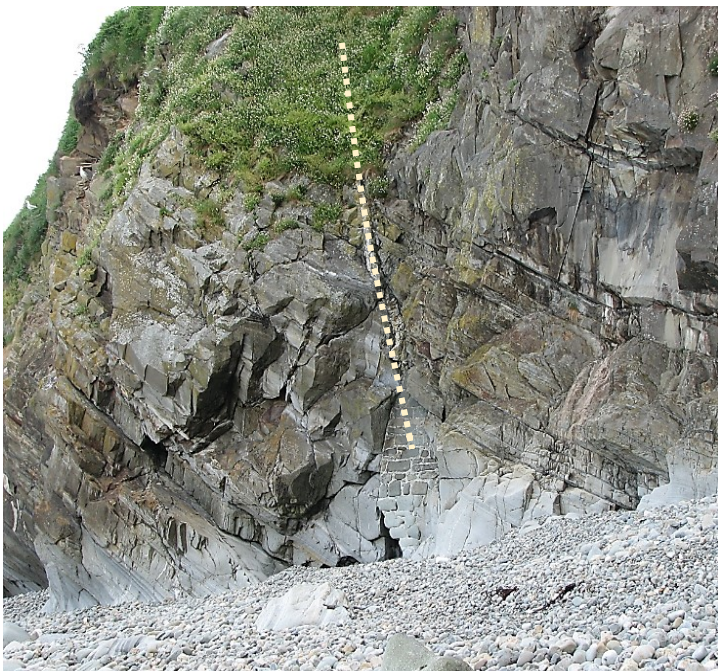
Figure 156: Clogau formation in the cliffs at Friog. The line of a fault is marked. Masonry infill has been used to reduce marine erosion along the fault line, protecting the railway at the head of the cliff.
